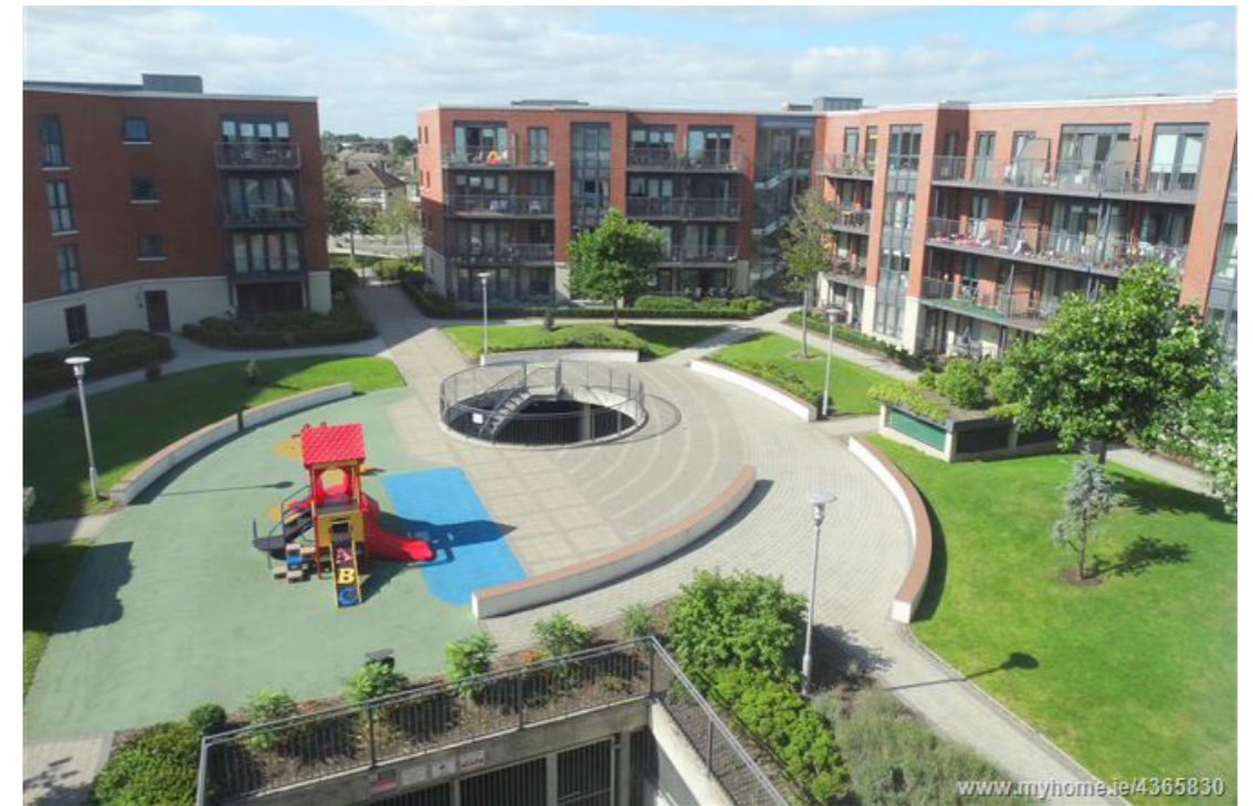
Figure 47. Indicative image of entrance to undercroft parking and landscaped communal podium above. Source: MCORM, 2022
